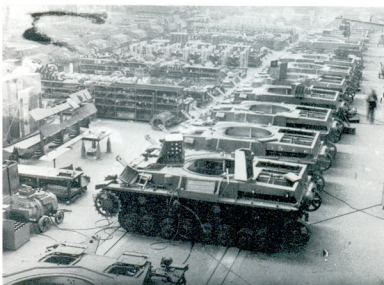
BW tanks on the assembly line in St. Valentin, Lower Austria. The ammunition racks can be seen on the tank in front.
