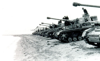
A Panzer IV company, obviously on going swimming. The photographs show the new one-piece cover of the commander's cupola that was used on all Ausf. H. ➡
