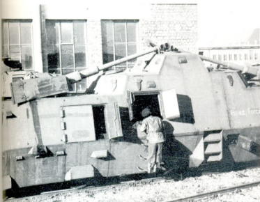
Armored trains and trolleys were also equipped with original Panzer IV turrets. Both short and long tank guns were used in them. The photograph above shows an armored trolley being shown to Hitler; below is an armored train, with two turrets, that was captured by the Allies.
