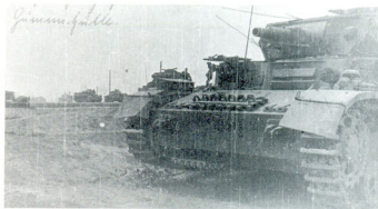
For Operation "Sealion", Panzer IV tanks were outfitted to travel underwater. This photograph shows such a vehicle in Russia in 1941. On its turret it still has attachment points for the rubber cover intended to make the turret watertight.
