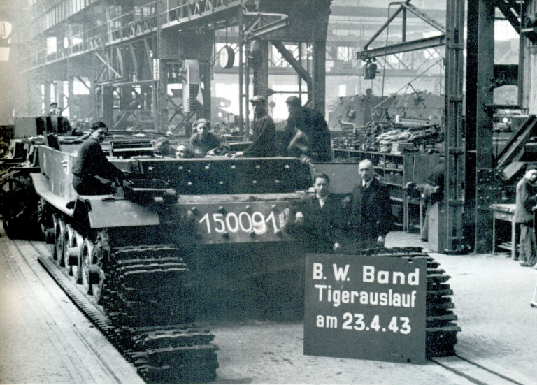
This photograph from the Nibelungenwerke shows the last Porsche Tiger chassis on the BW assembly line. Just behind it, full scale production of Panzer IV is underway.
