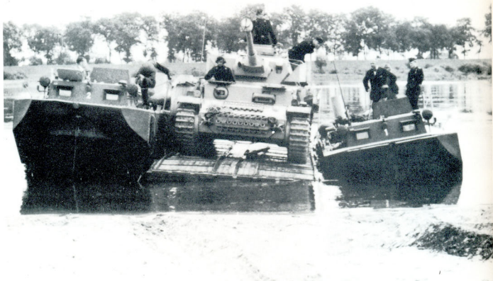
Two views of the Panzerfähre as it was originally used. A bridge capable of carrying loads of up to 24 tons was suspended between the two vehicles. The calculation of load weights was obviously insufficient, since situations such as that shown in the photograph occurred constantly. The lower photograph shows a prototype bridgelayer with six-roller running gear being ferried.
